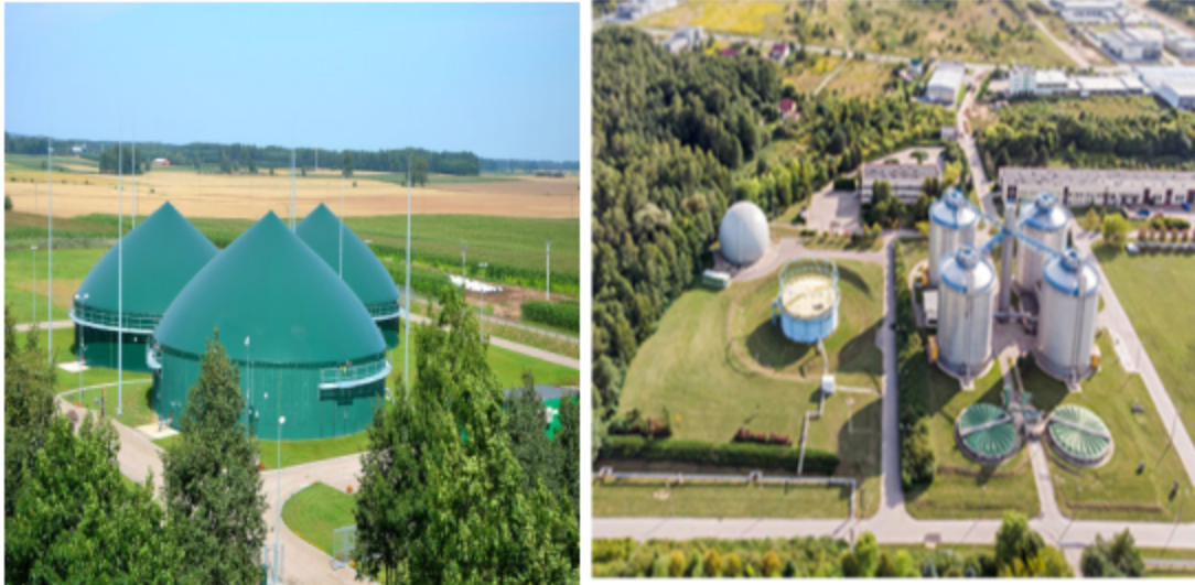
Figure 3: Biogas plants in Poland: (a) agricultural biogas plant (b) biogas plant in a sewage treatment plant [117]
