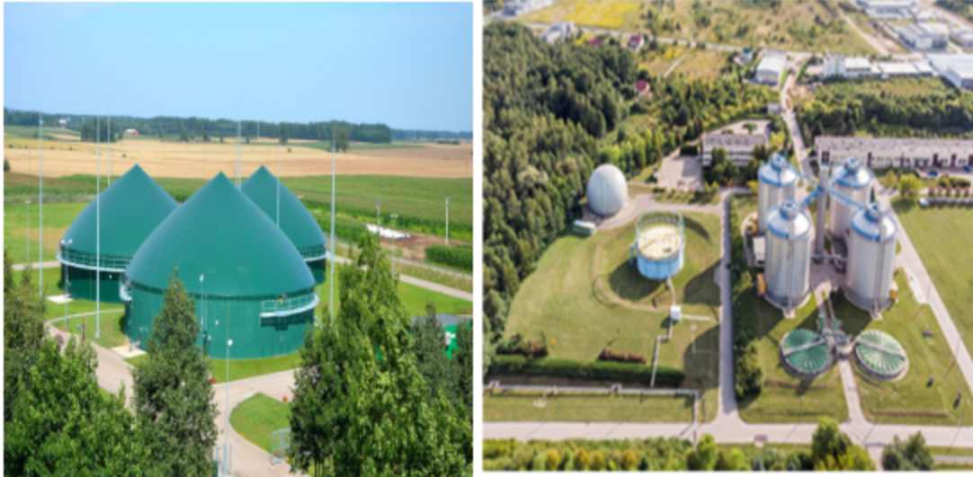
Figure 3: Biogas plants in Poland: (a) agricultural biogas plant (b) biogas plant in a sewage treatment plant [117]
